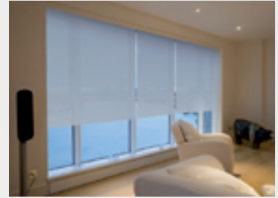
Motorised Blinds & Curtains
